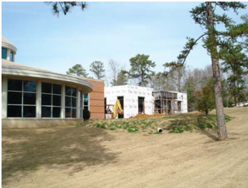
Auburn Public Library Expansion
